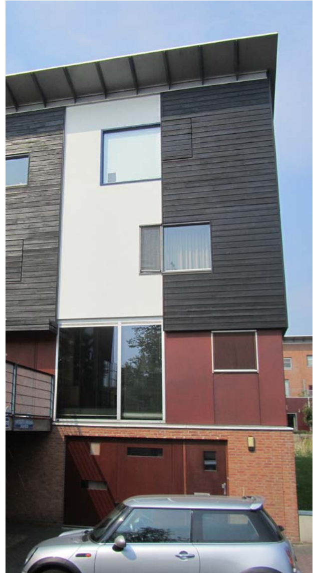
Cars are well integrated into the design of the scheme.
