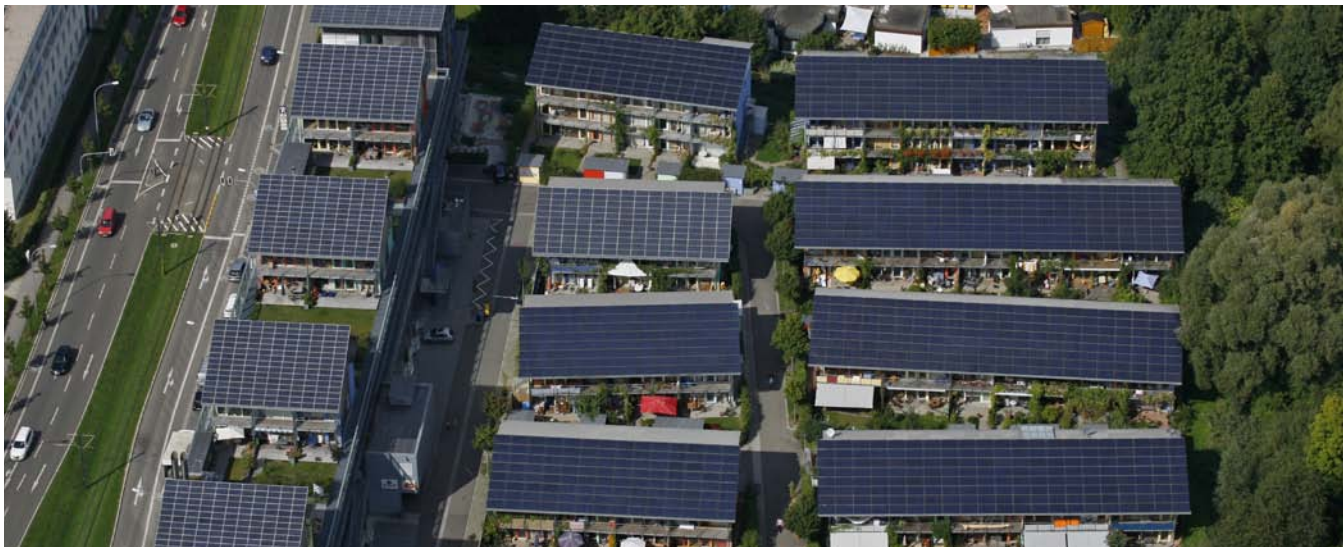
All houses are fitted with photovoltaic cells on their roofs.
