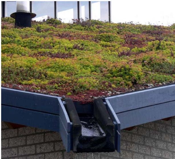
Eva Lanxmeer is filled with green-roofs and mirco-greenhouses.
