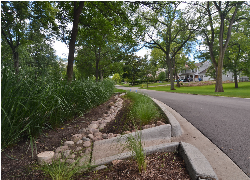
› Image 3 - A Bioswale, installations like this help the flow of stormwater which reduces the risk of flooding to homes and also recharges local aquifers.
