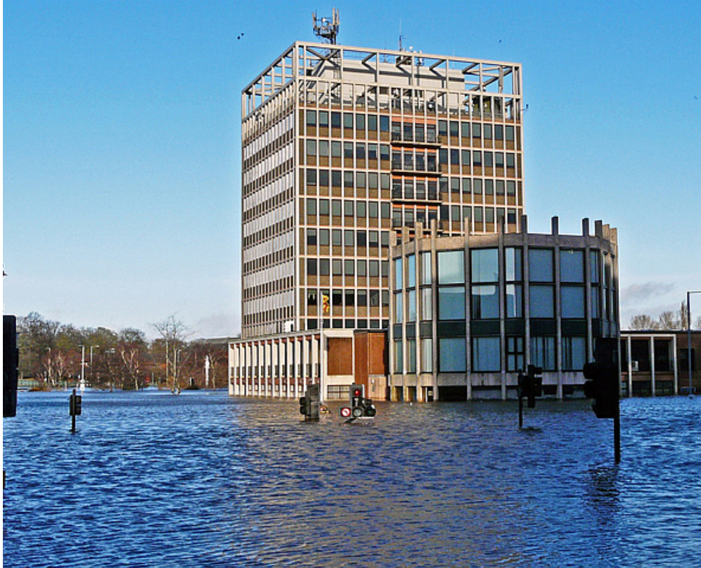
› Image 2 - Carlisle Civic Centre in the floodwater, December 2015. Ground floor was severely damaged.
