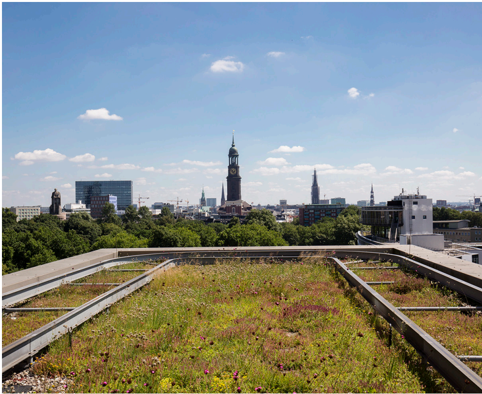
› Image 6 - Skyline of Hamburg, Germany, from a green roof
