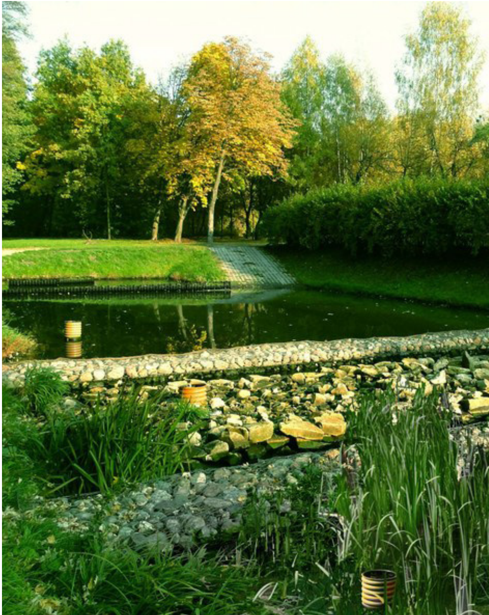
› Image 5 - Ponds and reservoirs built to reduce storm-water sewage flow peaks in Lodz, Poland
